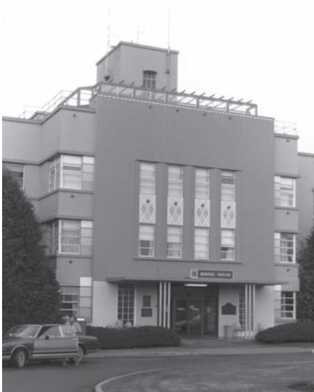
MEMORIAL PAVILION, ROYAL JUBILEE HOSPITAL 2355 Richmond Road Government of Canada Mercer & Mercer, Architects; 1947
