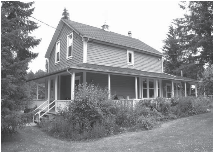
ERSKINE RESIDENCE 5323 West Saanich Road James Erskine, Owner; circa 1895
